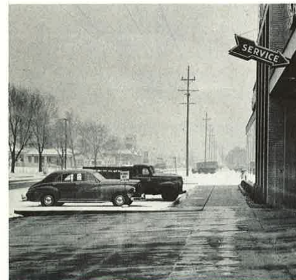
Figure 58: Pacific oil-fired boilers provide heat for the snow melting system protecting the concrete walk and driveway of Bennett Motor Co., Salt Lake City, Utah.
