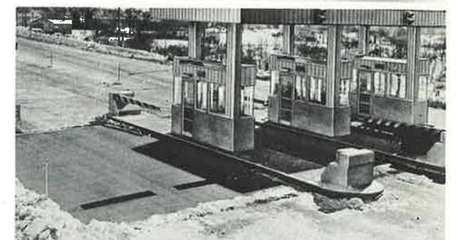
Snow melting system at the toll booths of the Raymond E. Baldwin Bridge, over the Connecticut River. Figure 41 (upper left) is a diagram of the pipe layout of this installation. Figure 42 (lower left) shows the project in the course of construction. Oil-fired boilers (Figure 43, top) can be expanded to take care of additional booths by simply adding more sections. Figure 44 (lower photo, above) shows cleared area, permitting easy stopping and thus reducing delay at booths.
