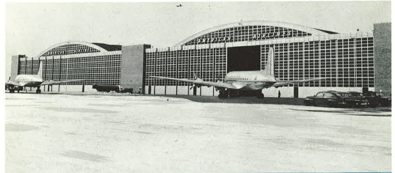
Figure 4 (above): Trackways for the heavy doors of the American Airlines hangars at the Chicago Municipal Airport
