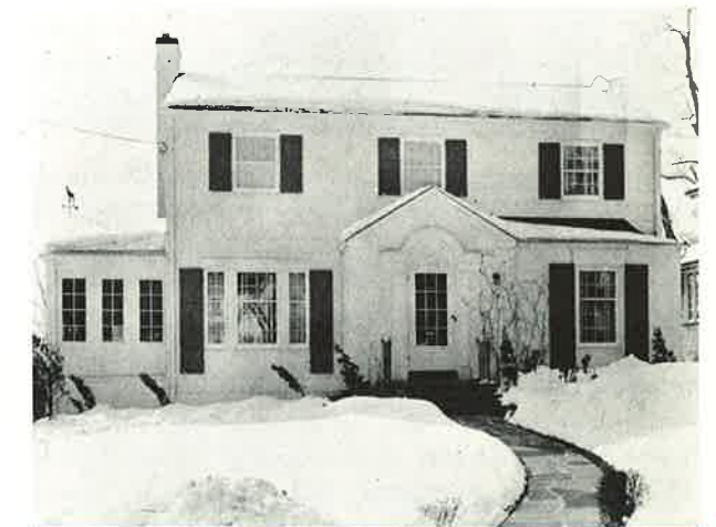
Figure 59: Coils buried in the steps and walk remove snow and prevent ice from forming. Installation is at the home of T. Napier Adlam, West Orange, N. J.
