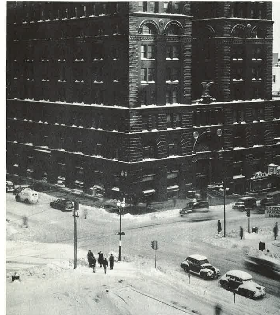
Figure 1: Snow and ice removal from the front and side walks of the Omaha National Bank Building, Omaha, Nebraska, is merely a matter of starting the snow melting system.
